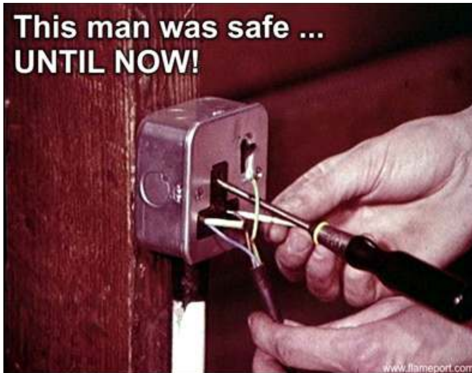
Fig 9.1.1.2: Example of a Potential Accident Area
