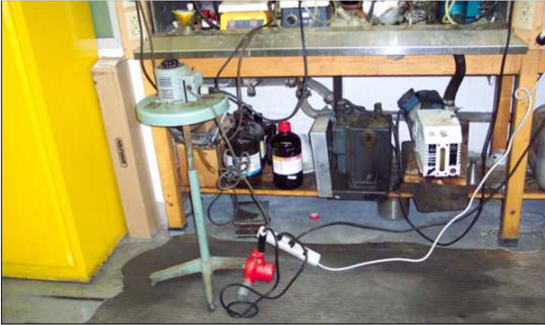
Fig 9.1.1.1: Example of a Potential Accident Area
